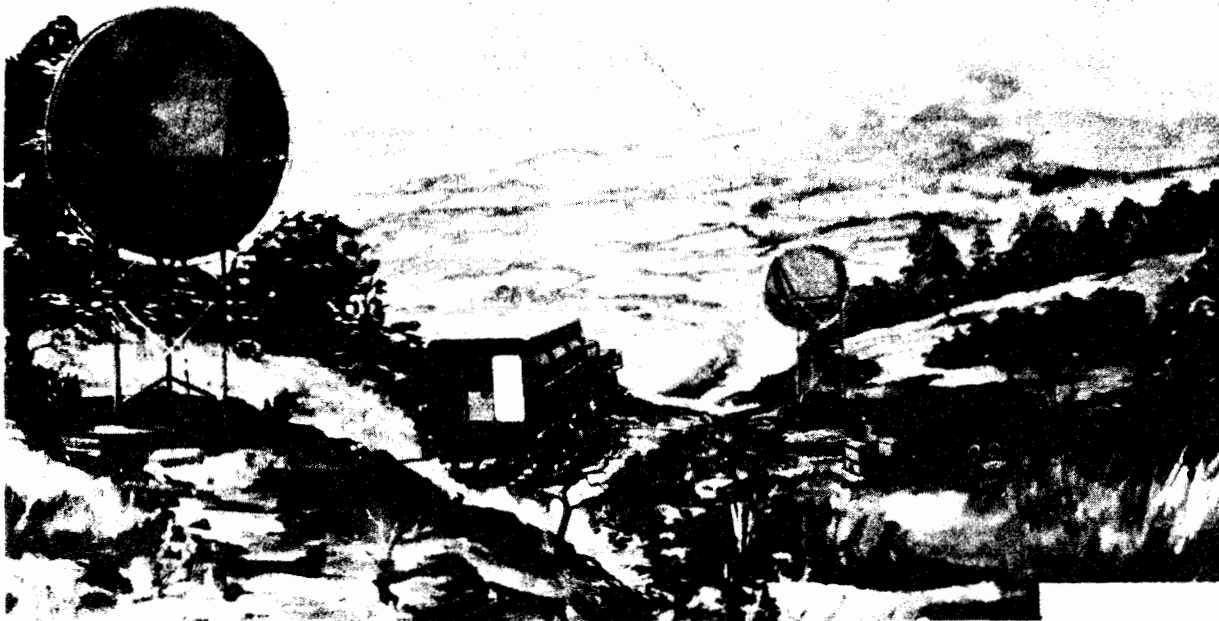
Typical AN/MRC-80 site
