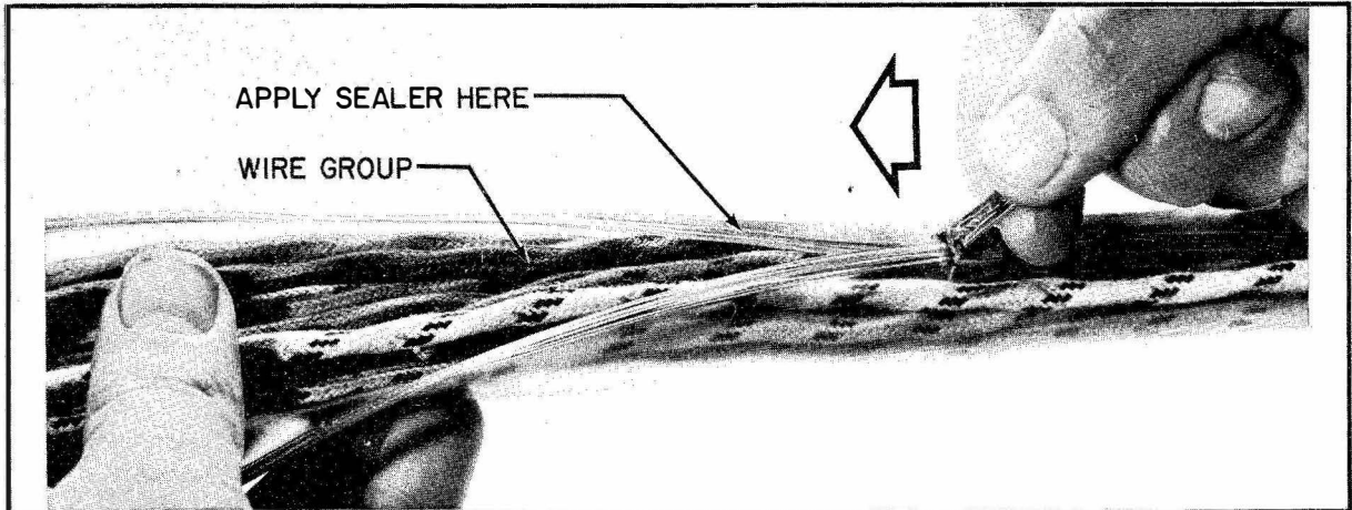
FIGURE 19-3 Installation of Zipper Tubing.
