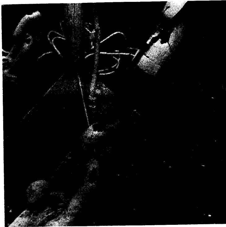
a. Mast Guy Turnbuckle and Shackles Figure 10-1. Typical Bonding Applications
