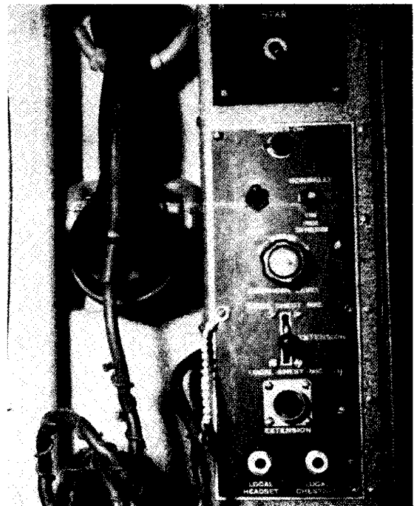
FIGURE 1.—A method of preventing failures of the hand-set cable of type 23972 radiophone unit.
