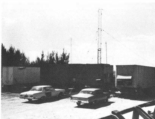
Receiver vans located on Naval Station serve as temporary radio receiving facility until the receiver site is established at Boca Chica Naval Air Station.
