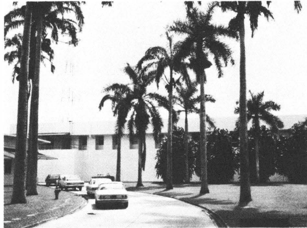
NAVCOMMSTA Balboa's headquarters and communication center.
