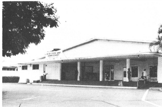
U. S. Army Commissary at Corozal.
