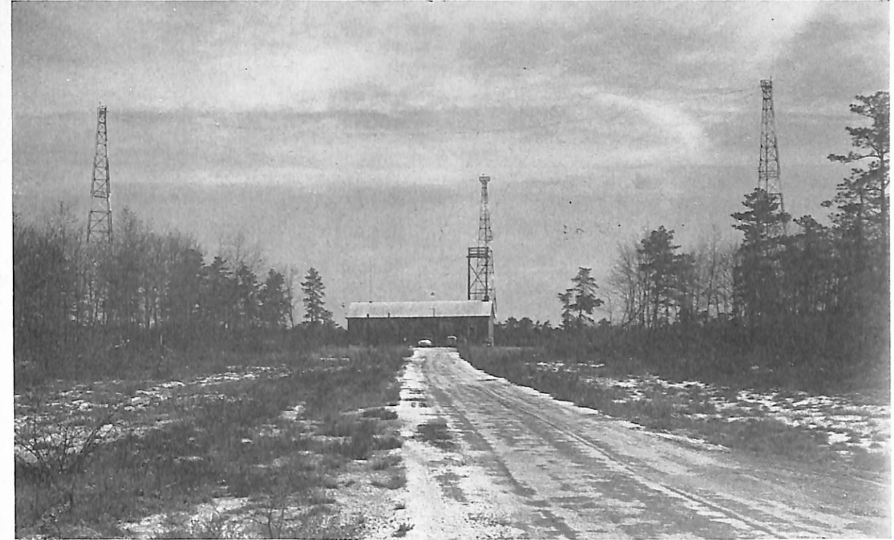
View showing vertical aspect of antennas. Six antennas on forward curtain are evenly spaced.
