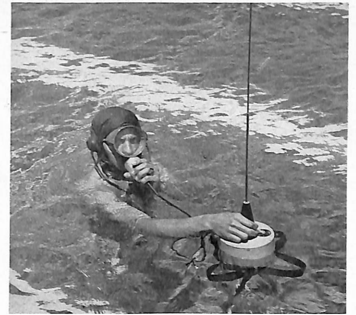
FIGURE 6—Swimmer sets switch on top of buoy and uses waterproof microphone to communicate with ship.
