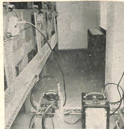
Model AN/PRM-1 connected to make a 24-hour period recording of radio interference intensities.
