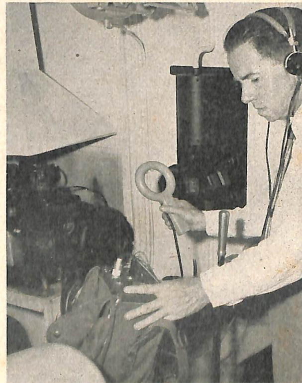
Detecting radiated interference from an auxiliary power supply aboard a 63-foot crash boat with the Eltron radio noise locator.
