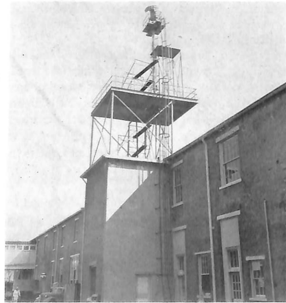
Tower Facility. Radio and Radar antennas installed here allow equipment testing under actual working conditions.
