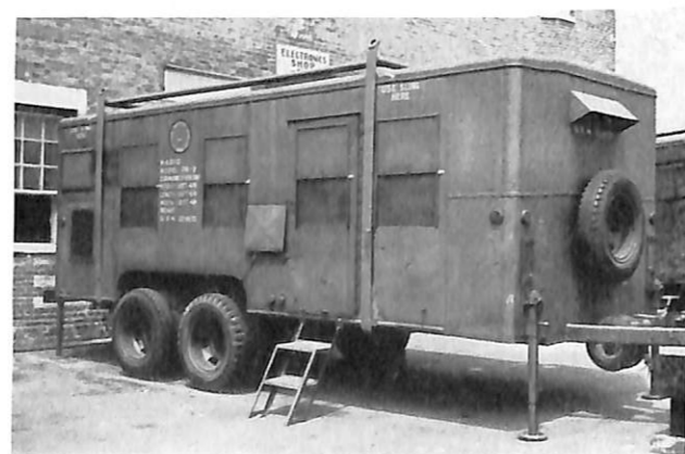
Mobile communication van, Model PN-2 U. S. N. 226639. Showing hoisting straps and new body constructed at the Norfolk Naval Shipyard.
