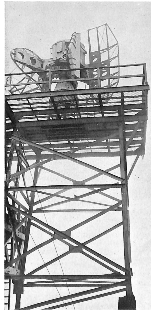
SX antenna platform atop Navy Building.
