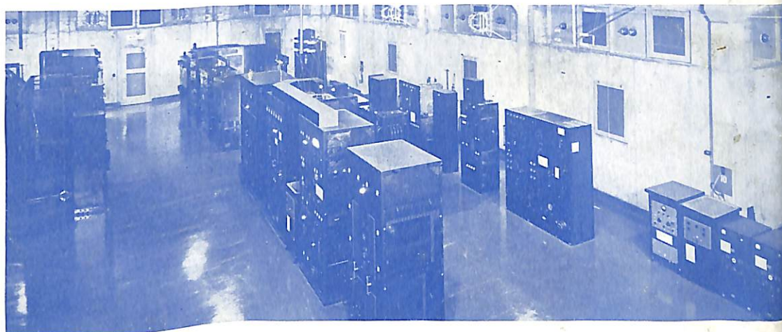
WING "A" FROM ROOF OF CONTROL ROOM
