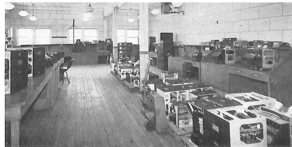
FIGURE 1—South end of G. C. A. maintenance shop.
