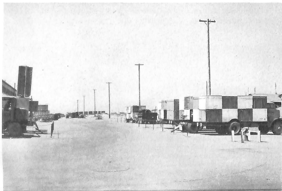
FIGURE 3—Parking area adjacent to G. C. A. maintenance shop.
