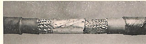
FIGURE 4—Copper sheet formed and soldered to the copper braid.
