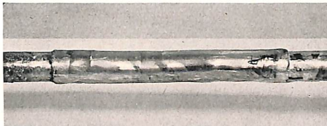
FIGURE 9—Second lead sleeve soldered in position over the first lead sleeve.
