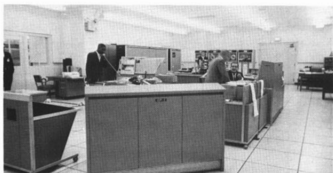
Above: AUTODIN operations area at NCU Albany, N. Y.
