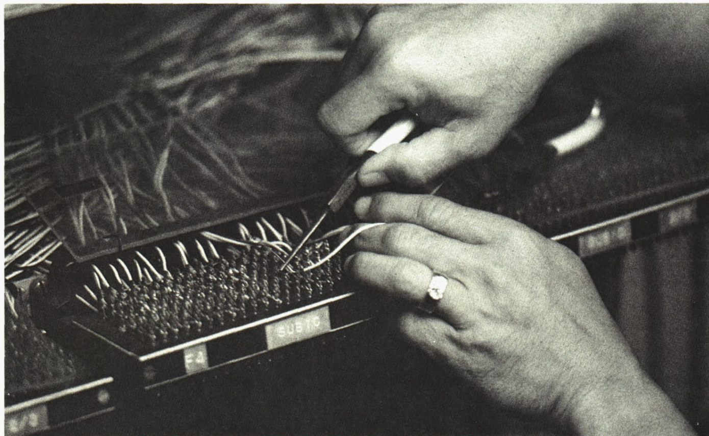
Hundreds of thousands of cross connection panels meshing communication facilities in the area are housed on the fourth deck of the link station.
