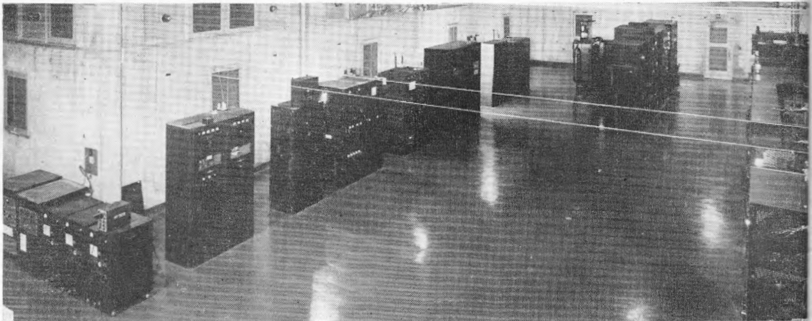
WING "C" FROM ROOF OF CONTROL ROOM
