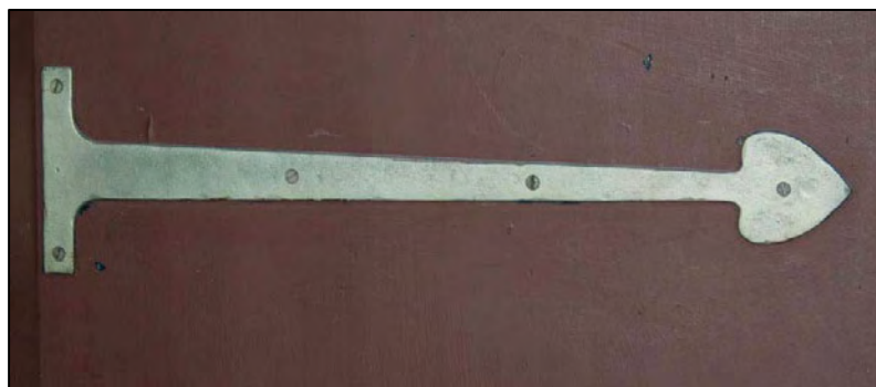
Figure 53b. Extant reproduction strap hinge on Northeast Pavilion entrance door, D108. Note the similarities to the hardware in the catalog illustration.
