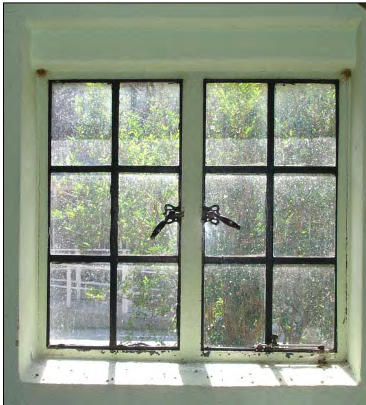
Figure 36. Power House, SE elevation, interior elements of window opening, 2008.
