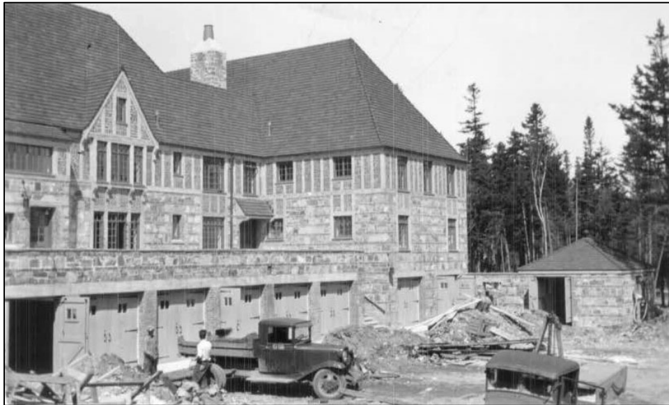
Figure 14. Apartment Building, SE elevation depicting completed exterior of building and debris removal, September 15, 1934.
