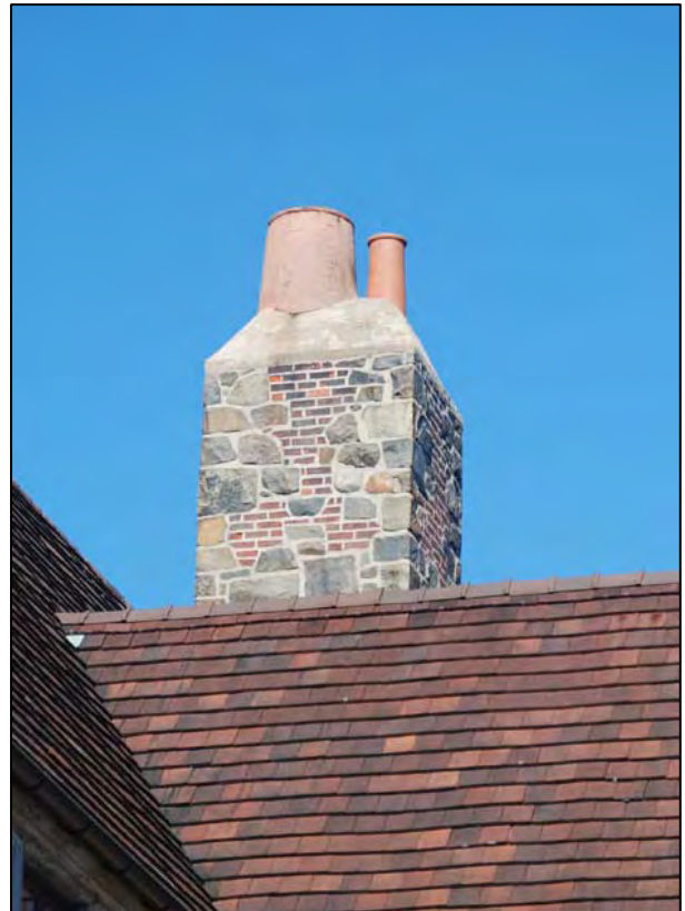
Figure 55. Apartment Building, SW chimney, 2008.
