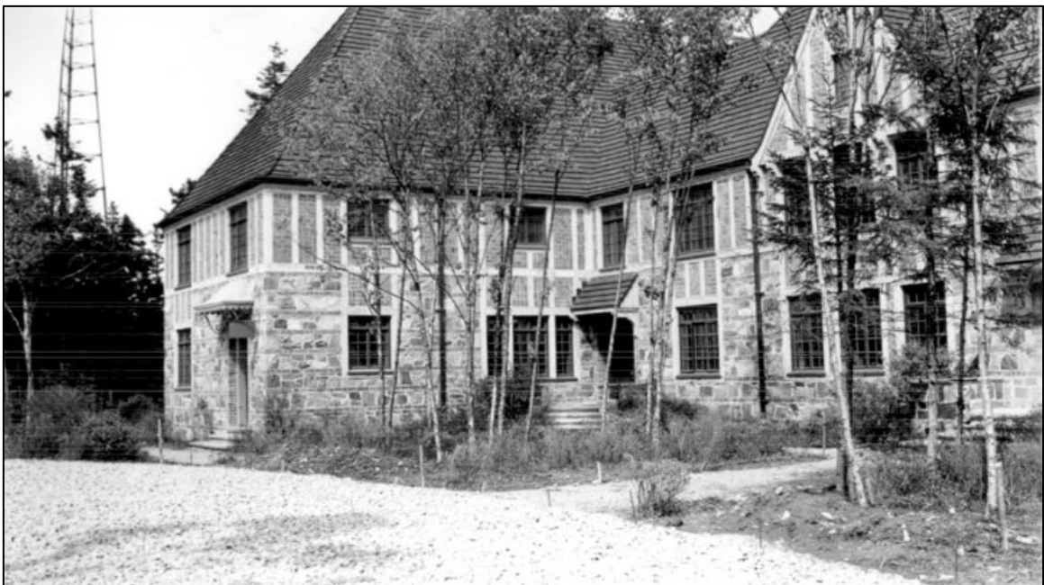
Figure 18. Apartment Building, NW elevation courtyard depicting some scrub cleared, shrub planting completed, driveway and paths graded, and graveled, seeding and cleanup still required, June 1935.
