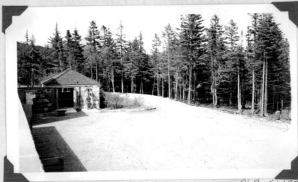
The same view in June, 1935, after the curb had been installed and planting partially completed at the end of the court. Planting must still be done around the court, and cleanup has not been begun.
