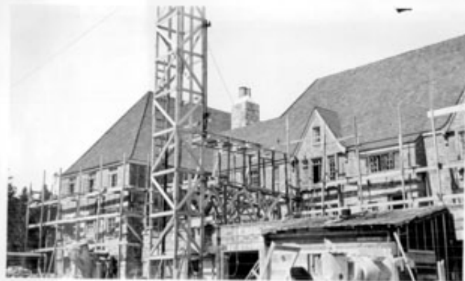
Apartment Bldg. S. E. side
