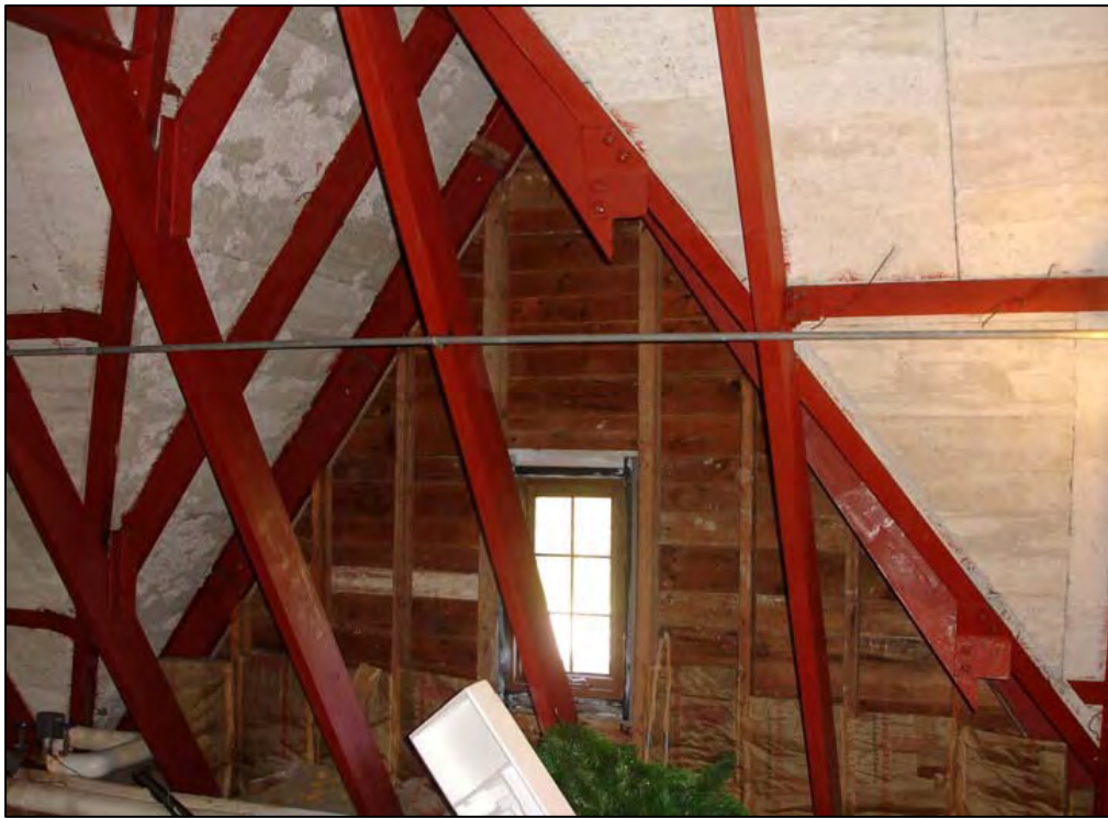
Figure 69. Apartment Building, attic story, typical framing of roof and cross gable, 2008.
