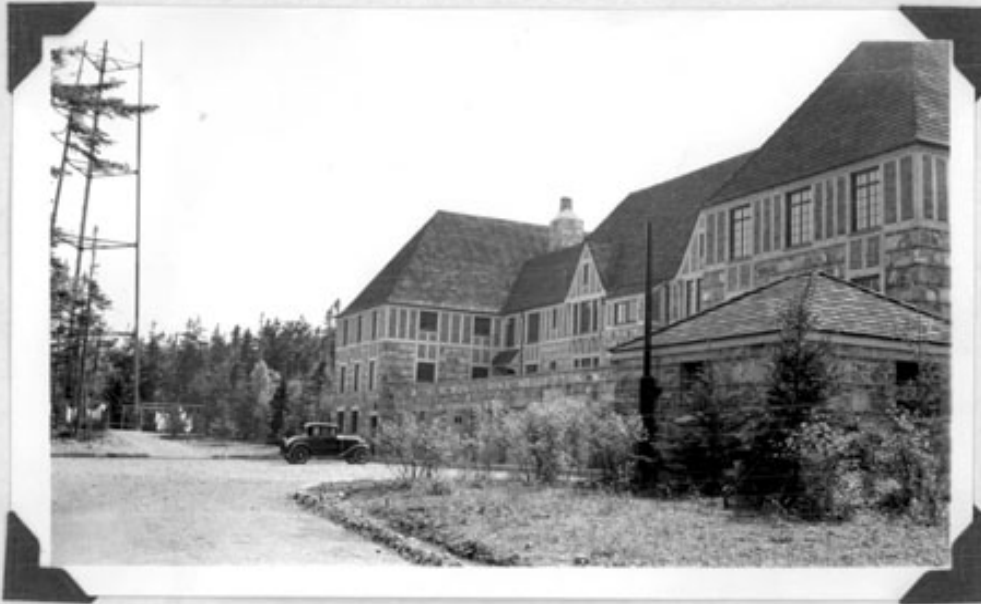
The Radio Apartment Building from the service court entrance, June, 1935. Surfacing of drive and court, finish grading, seeding and some planting and cleanup work has still to be done.
