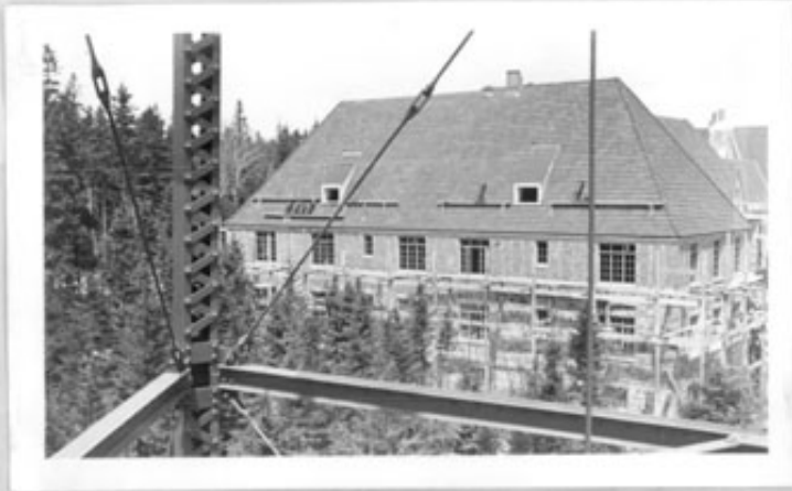
Apartment Bldg. S.W. Side
