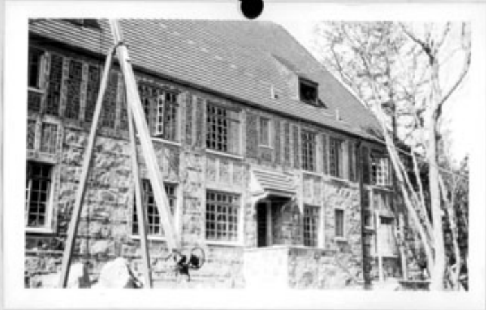
Apartment Bldg N.E. side
