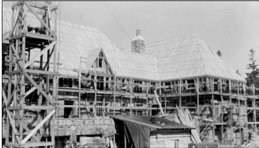
Figure 13. Apartment Building, SE elevation, April 14, 1934.
