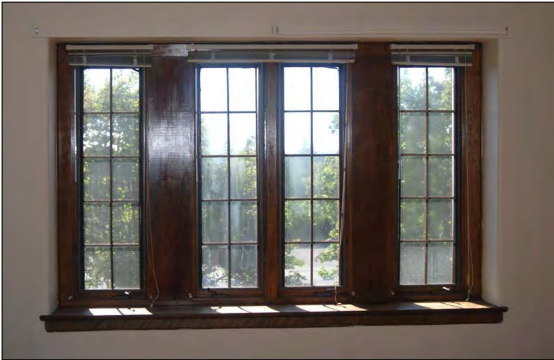
Figure 63. Apartment Building typical interior of window opening with four sashes (W237), 2008.
