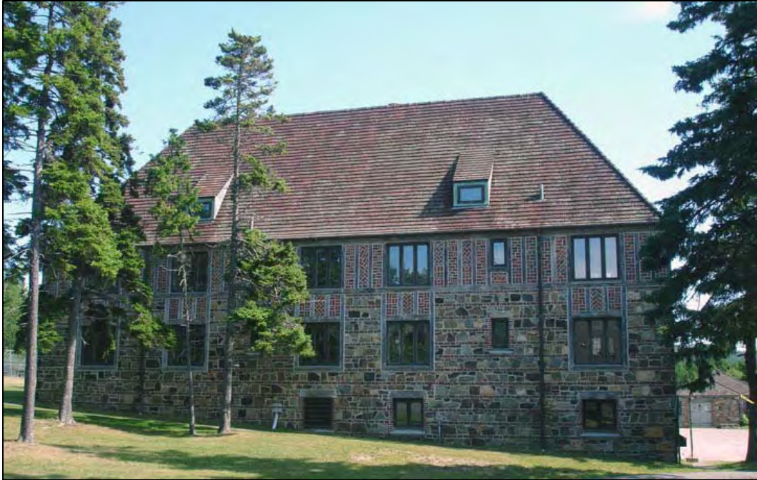
Figure 46. Apartment Building, SW elevation, 2008.
