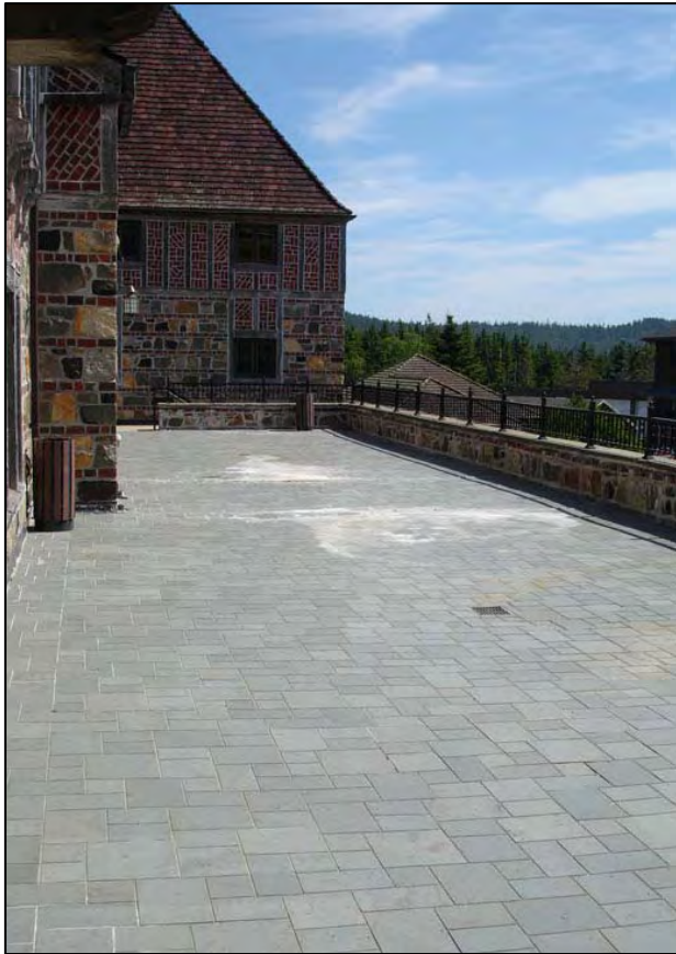
Figure 51. Apartment Building, SE elevation, terrace, 2008.
