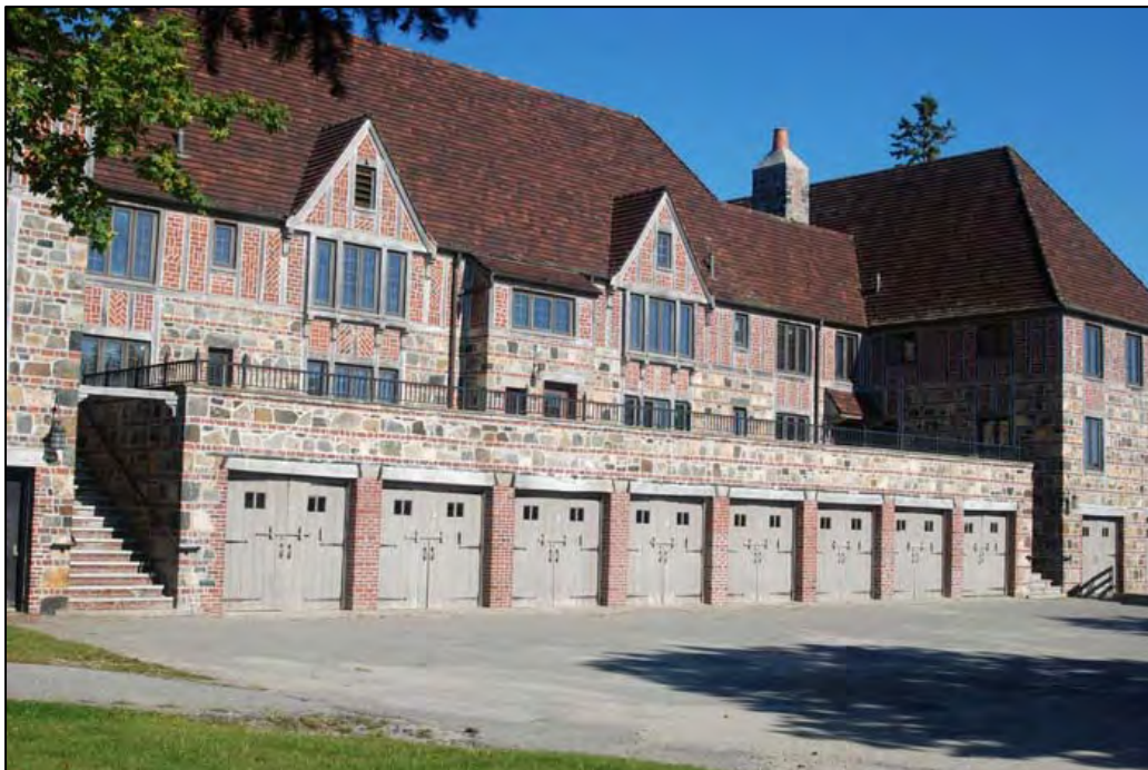
Figure 44. Apartment Building, SE elevation depicting garage bay doorways at basement story, 2008.
