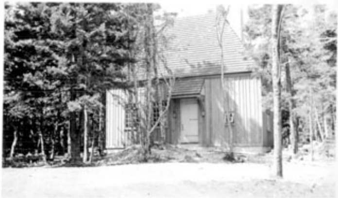
Intercept Bldg from S. E.
