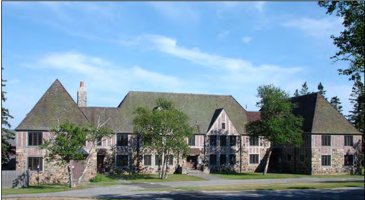
Figure 39. Apartment Building, NW elevation, 2008.
