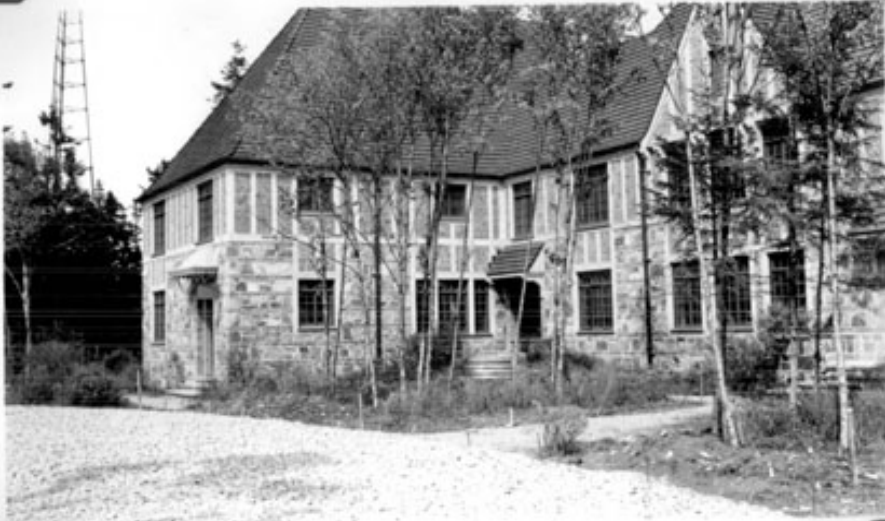
P67 55 of 73 The same corner with shrub planting completed, but surfacing of drives and paths, seeding, and cleanup work still to be done.
