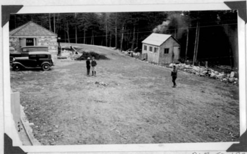
The service court after drainage and sub-grade had been completed in November, 1934.
