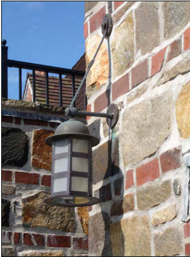
Figure 56. Apartment Building, SE elevation, exterior light fixture on Northeast Pavilion, 2008.
