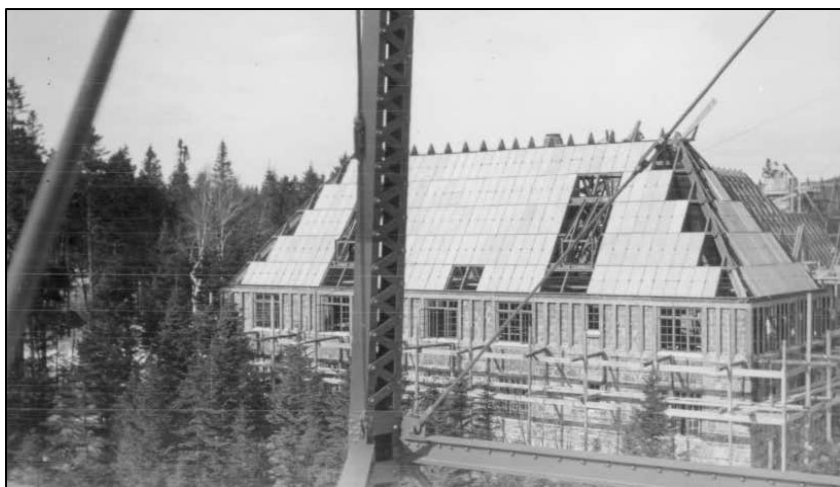
Figure 12. Apartment Building, SW elevation, March 8, 1934.
