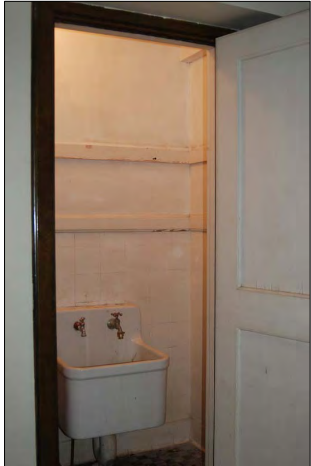
Figure 62. Apartment Building, NE Hallway utility closet, 2008.
