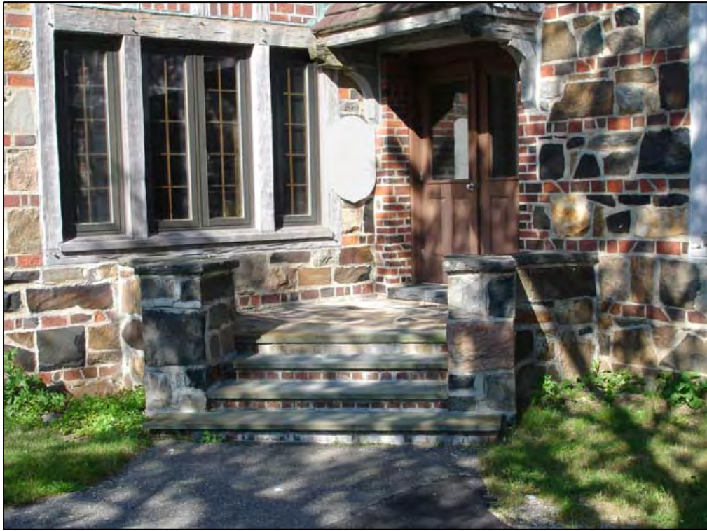
Figure 49. Apartment Building, NW elevation entry stoop to D102, 2008.
