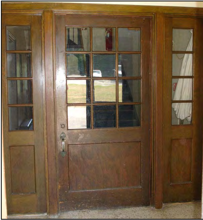
Figure 61. Apartment Building, Center Hallway NW vestibule interior doorway, 2008.
