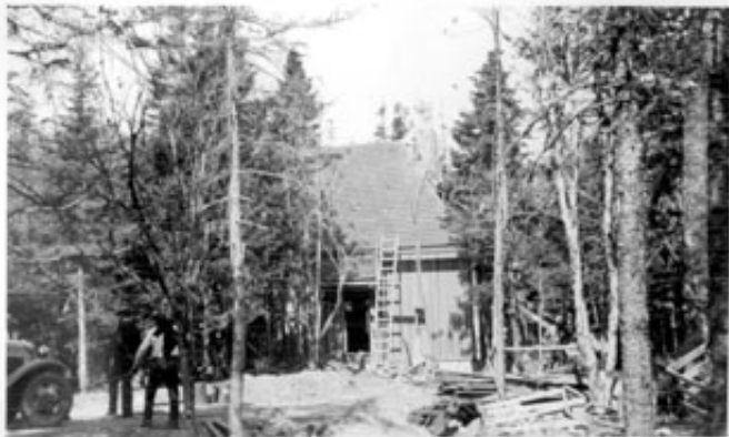
Intercept Bldg. From S. E.
