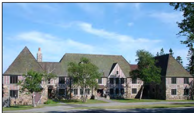
Figure 2. Apartment Building, northwest (NW) elevation, 2008.
