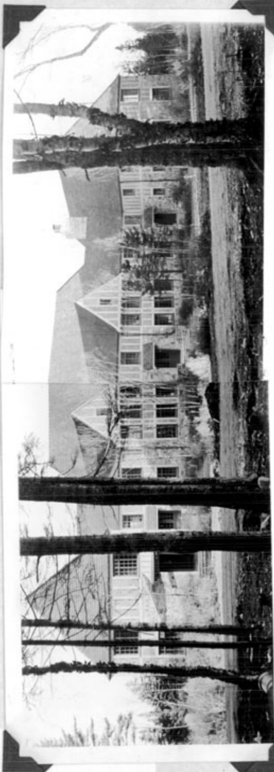
Panorama showing the Radio Apartment Building as it was in November, 1934, after planting had been partially completed. Subgrade of driveways and paths is in place, loam has been placed in planting beds and areas to be seeded.
