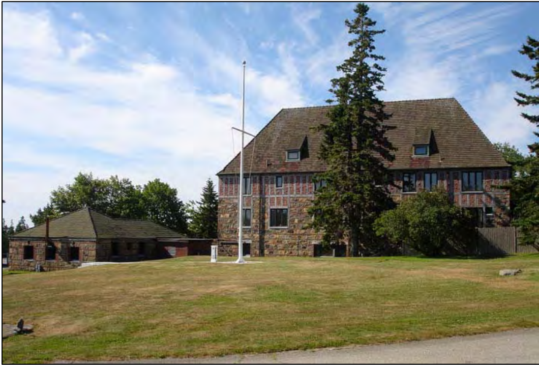
Figure 45. Apartment Building, NE elevation with Power House on the left, 2008.
