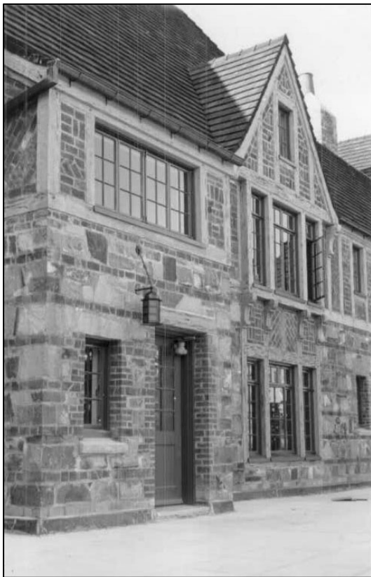
Figure 21. Apartment Building, SE elevation, center bay and cross-gable bay, September 1934.
