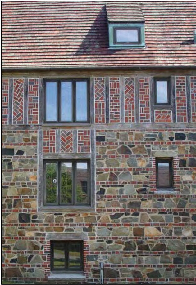
Figure 54. Apartment Building, SW elevation, window openings depicting exterior elements of different window types including: Basement, W002 (type C); First Story, W120 (type G), W121 (type A, masonry surround); Second Story, W224 (type G), W225 (type A, wood surround); Attic, W304 (type J in dormer), 2008.
