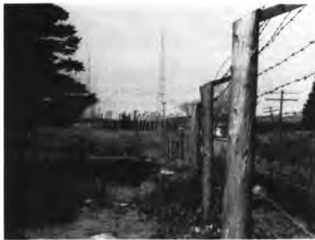
Barbwire security fence, Otter Cliffs. Note telegraph pole line at right and antenna towers in distance. Photo courtesy Carl Herr.
