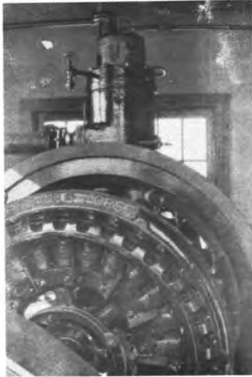
NBD - Radioman Ted Hancock's "Pride & Joy" -- The Standby power plant at Seawall !
