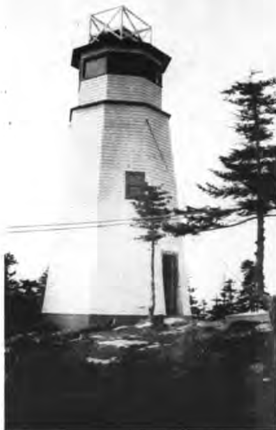
Otter Cliff lookout tower. It became NBD Radio Compass Station after the war. Photo courtesy Carl Herr.
